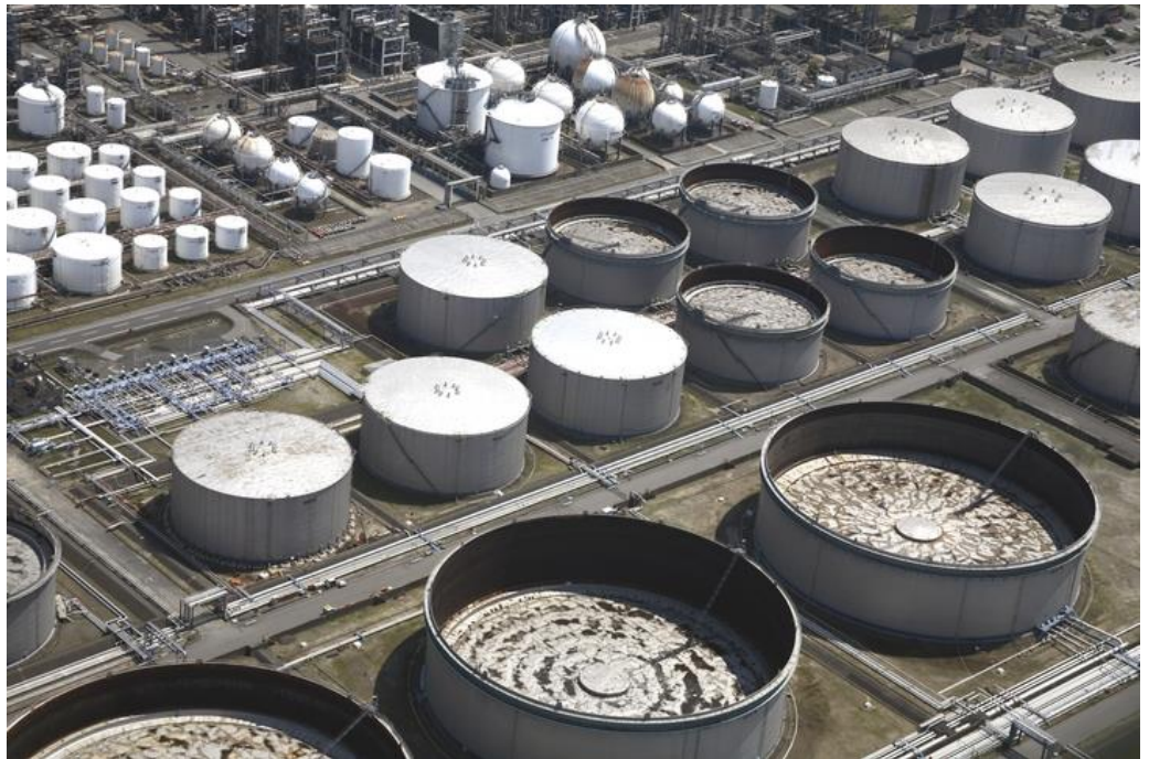
A petrochemical complex (Photo courtesy of AFLO)
