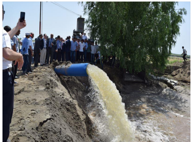
Water pumping to the canal
