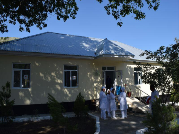
Medical point constructed by the project
