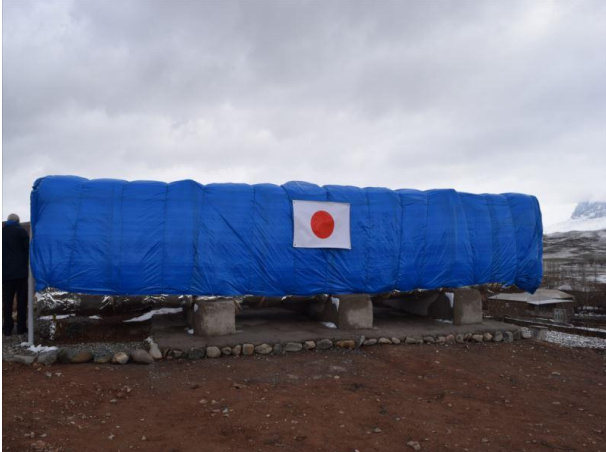
Water tank constructed by the project
