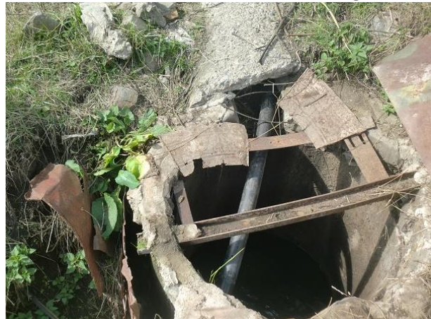
Broken water collector in the village
