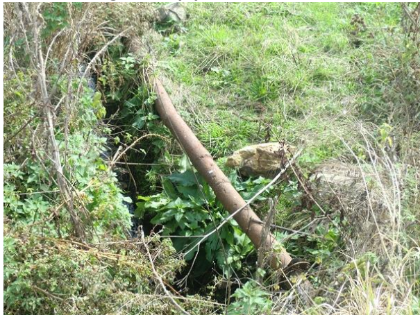
Rusting water pipe which is unusable
