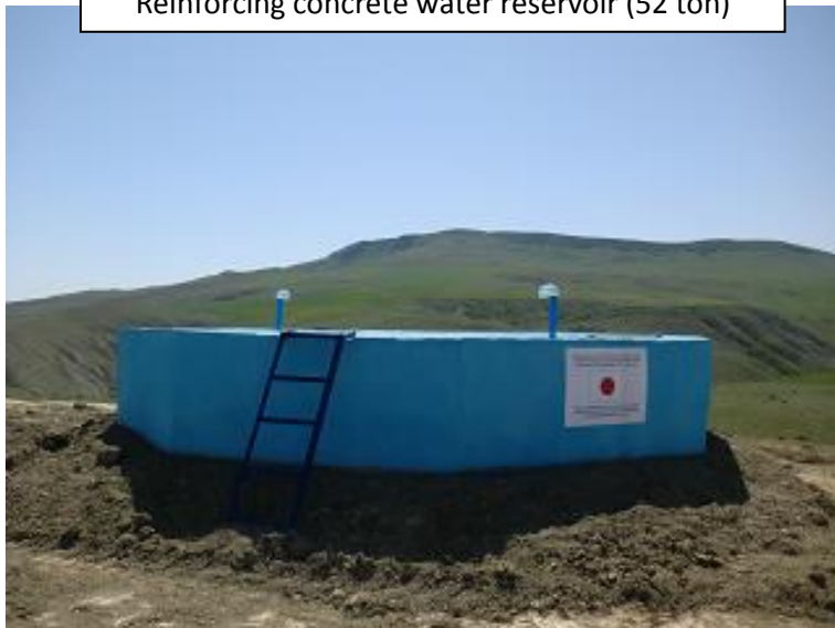
Reinforcing concrete water reservoir (52 ton)
